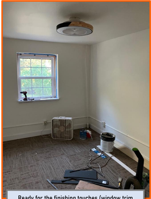
Ready for the finishing touches (window trim particularly).
