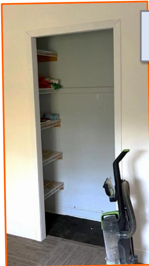
The new trim scheme of door casing and baseboards mimics existing original examples in the closet – as close to the room's 1928 appearance as it's been in years.
